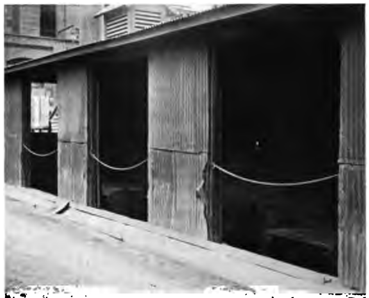
Fig. 4. Doorways protected by chains.*
